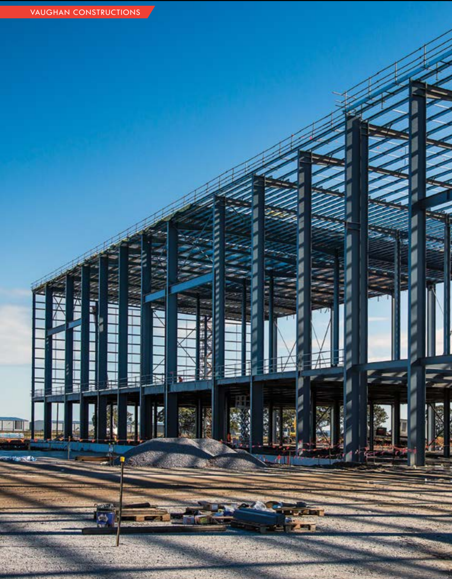
Woolworths Merinda Village Shopping Centre Under Construction, Victoria
